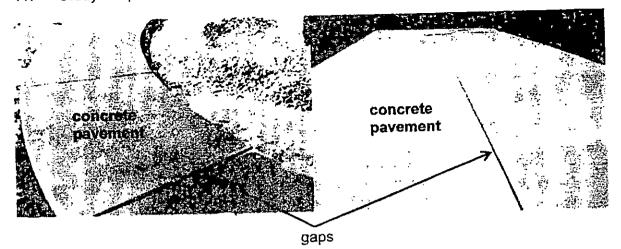
(a) These concrete pavements were purposely built with gaps in between.
